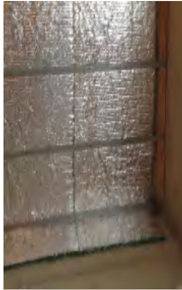
Basement Wall Cavity
